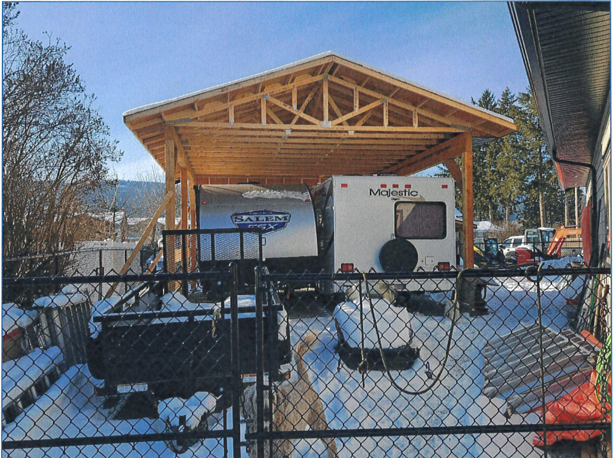
Figure 3: Accessory Residential Building at 159 Riverdale Drive
